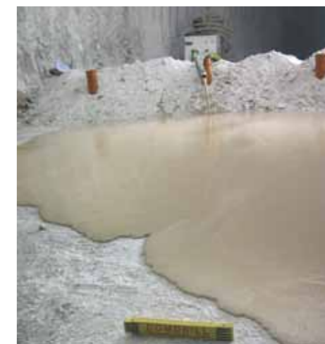
Pumping of concrete backfill at Asse Mine (Germany)
