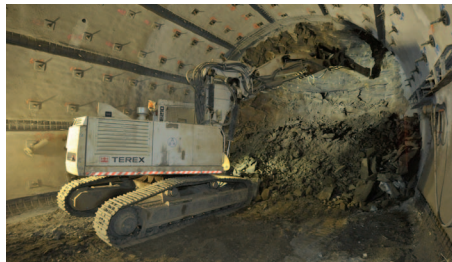
Construction work in Jurassic marls. Konrad repository (Germany).
